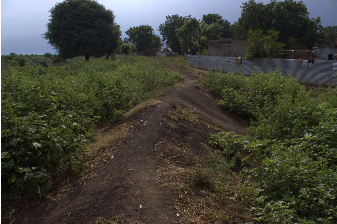
Figure 8: Earth terrace in Afrush Tobak village built in 2022 to protect the village from the flood.
